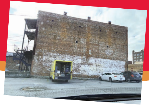
Wall of Jennison Building 410 N Main Street
